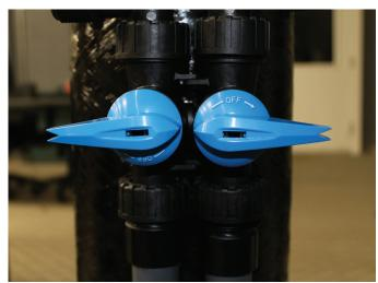
1. Turn both handles on bypass to bypass position (horizontal with the plumbing).
